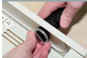
FLP conduit with sheath trimmed back
